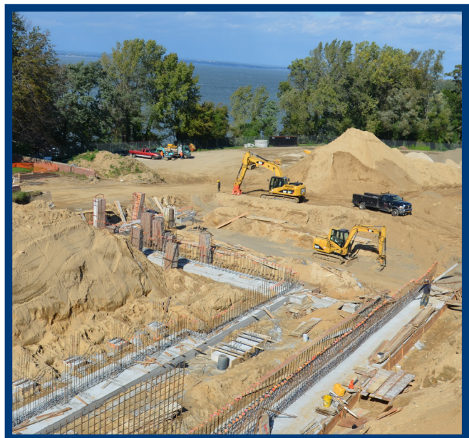
Construction of the lower level during October 2018
