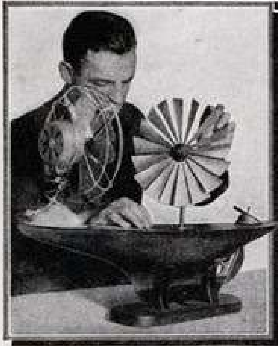
Air blast from fan turns windmill mounted on model boat, in demonstration at English inventor's exhibit. At right is artist's conception of ocean liner using the wind-propeller sails.
