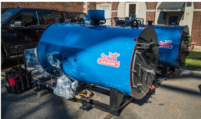
New Boilers awaiting installation
